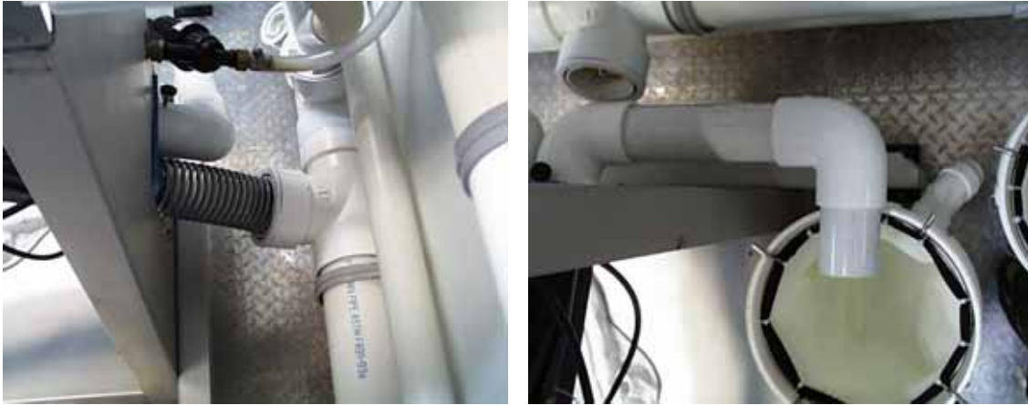
Figure 49: Line Isolation Port Installed
